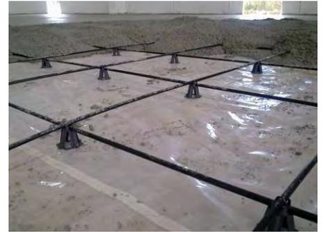
*The post-tensioned system that is usually used for slabs can also be applied to carry out industrial floors, thus allowing the floor industry to also take advantage of this technology.*
