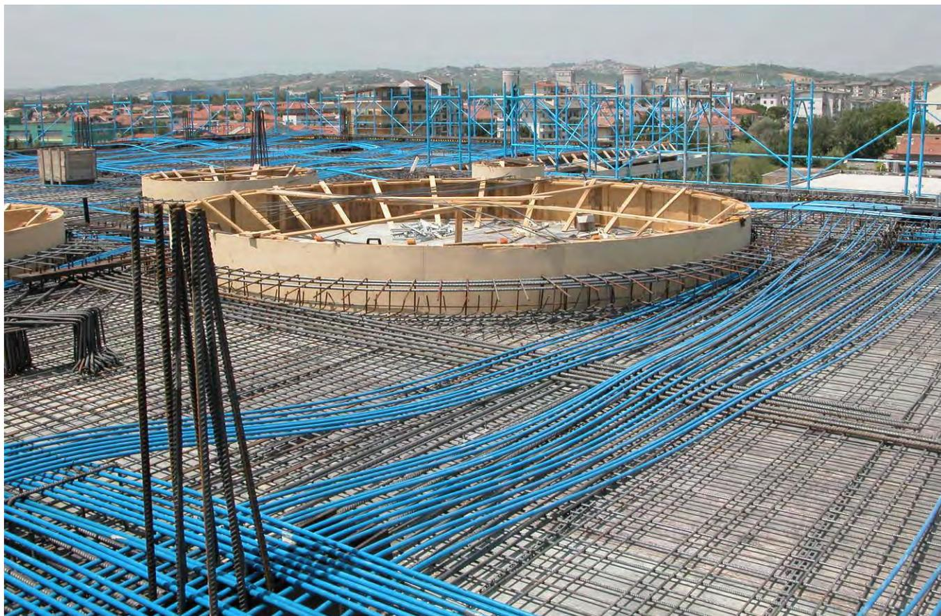
*The deformation and crack control are some of the aspects that are effectively controlled by the application of cables, in spite of the conventional reinforced concrete structures.*
