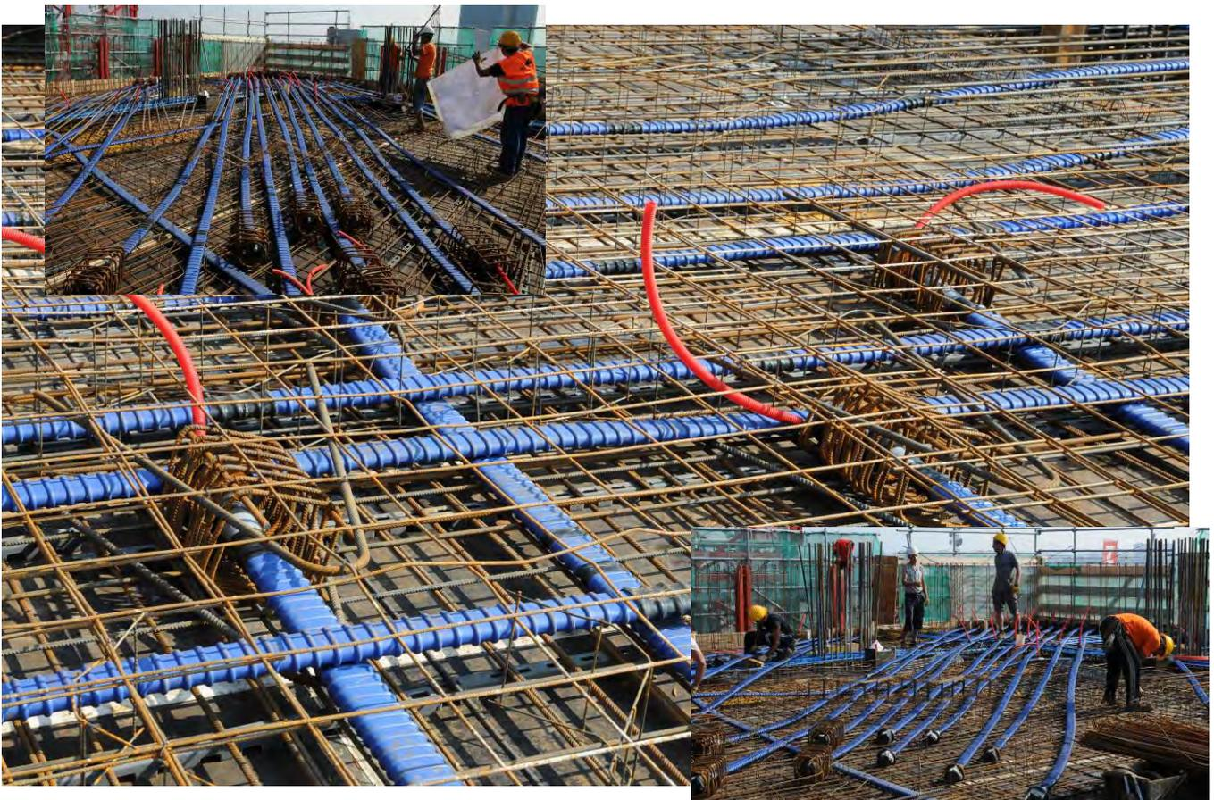
*Cables for bonded slabs may be supplied directly from factory rolled up with a diameter of 2.2 m, with the passive anchorage preblocked at one end and with sheaths.*
