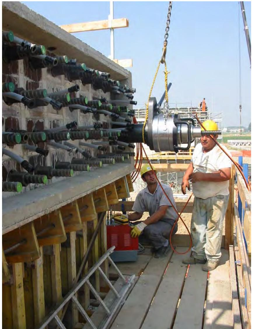
*Bar tensioning of diam. 40 mm with DD2000KN jack and TTM250-A pump*
