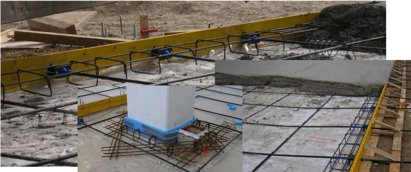
*Strands are inserted into the grouting delimitation formwork. According to the project indications, strands are positioned in parallel at a distance between 0.8 and 1.2 m. The project shall define:*
