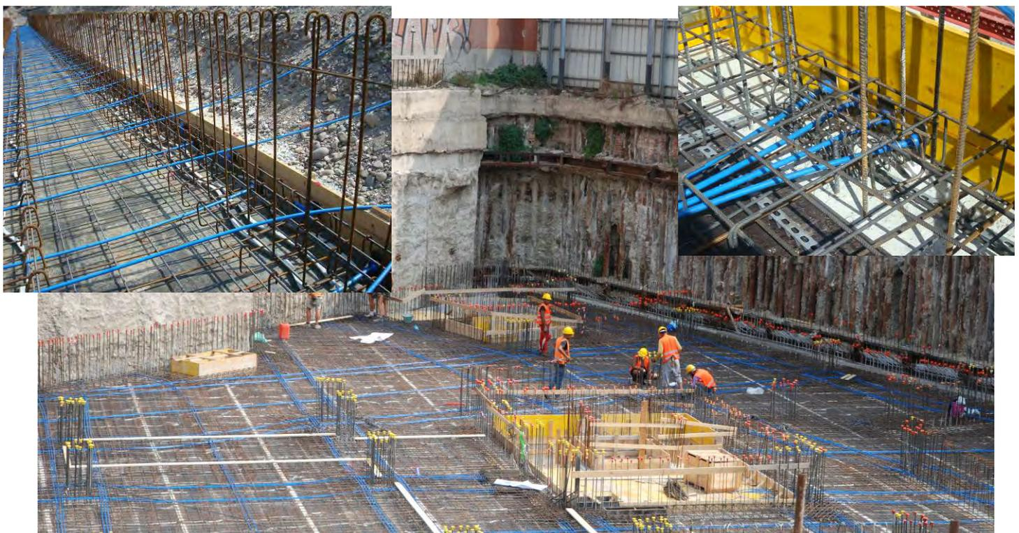
*Cables for unbonded slabs may be supplied directly from the factory rolled up with a diameter of 2.2 m, with the passive anchorage preblocked at one end.*
