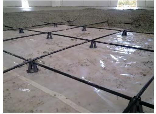
*The post-tensioned system that is usually used for slabs can also be applied to carry out industrial floors, thus allowing the floor industry to also take advantage of this technology.*
