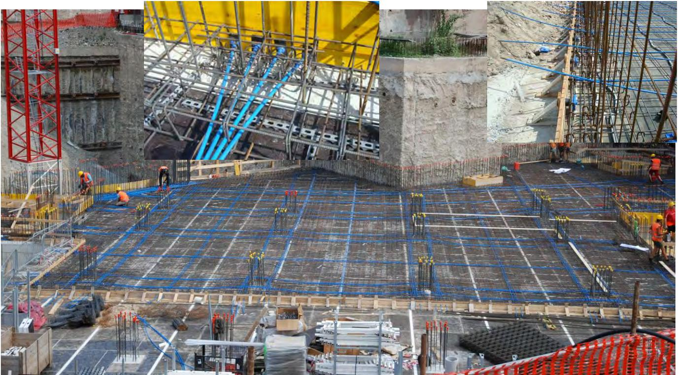
*The unbonded application is surely the most performing one, since it is protected against corrosion by both a grease and a polyethylene barrier. It requires no grouting after tensioning but a very accurate infilling (sealing) of the heads. In this application the load will always remain totally concentrated on the anchorage, therefore the sealing completes the protection of the anchorage over time and its importance increases together with the anchorage exposure to corrosion.*
