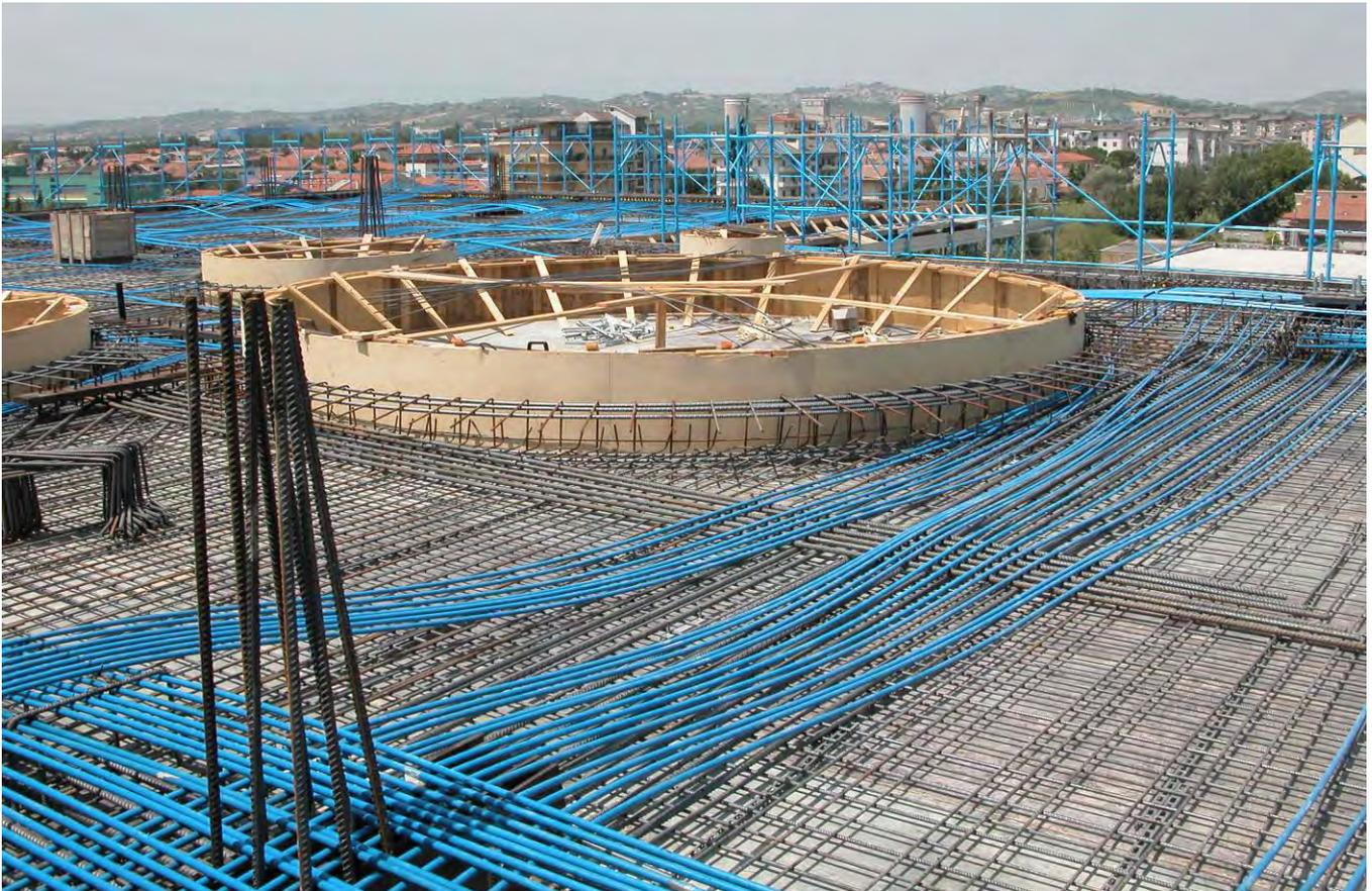
*The deformation and crack control are some of the aspects that are effectively controlled by the application of cables, in spite of the conventional reinforced concrete structures.*
