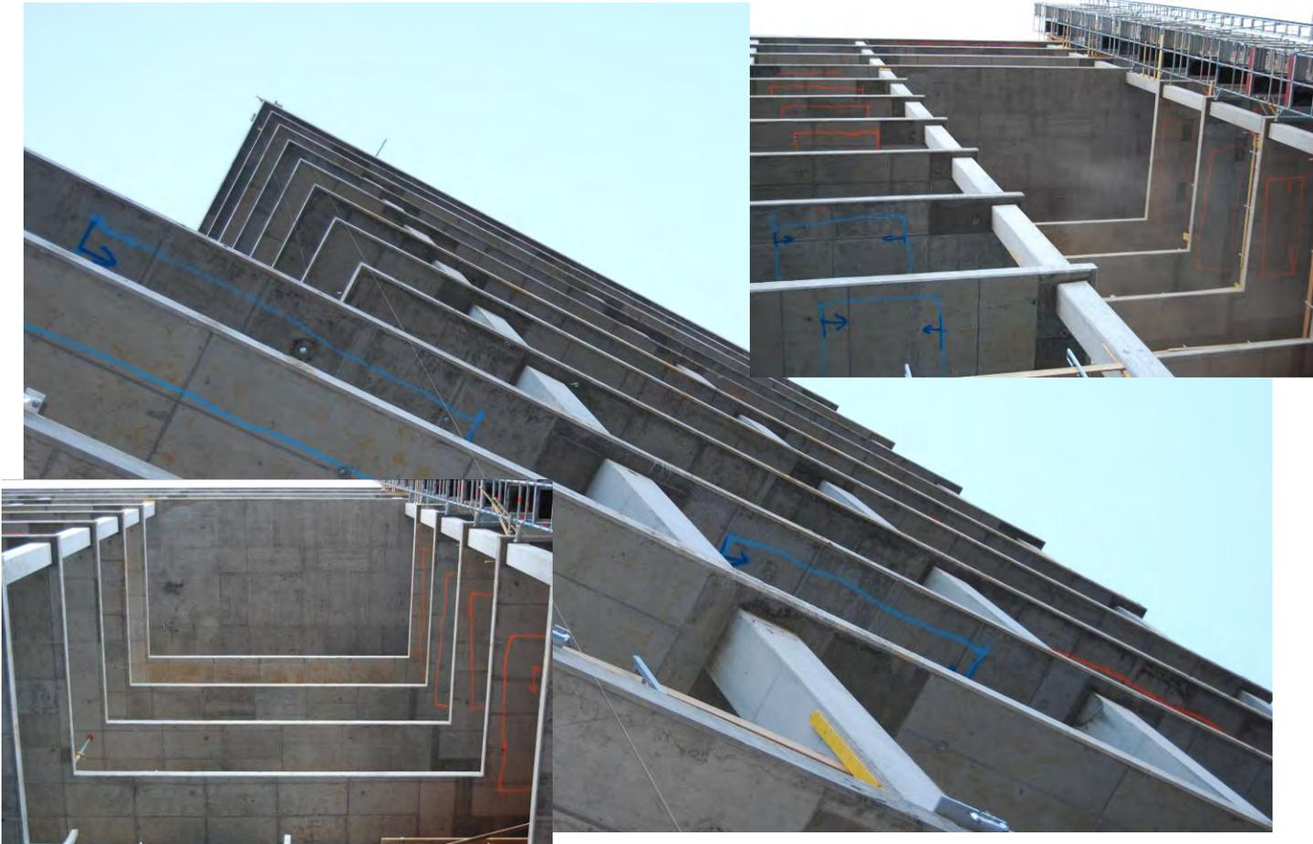
*Post-tensioning is very favourable in the construction of rectangular slabs with 8-12 m long sides.*
