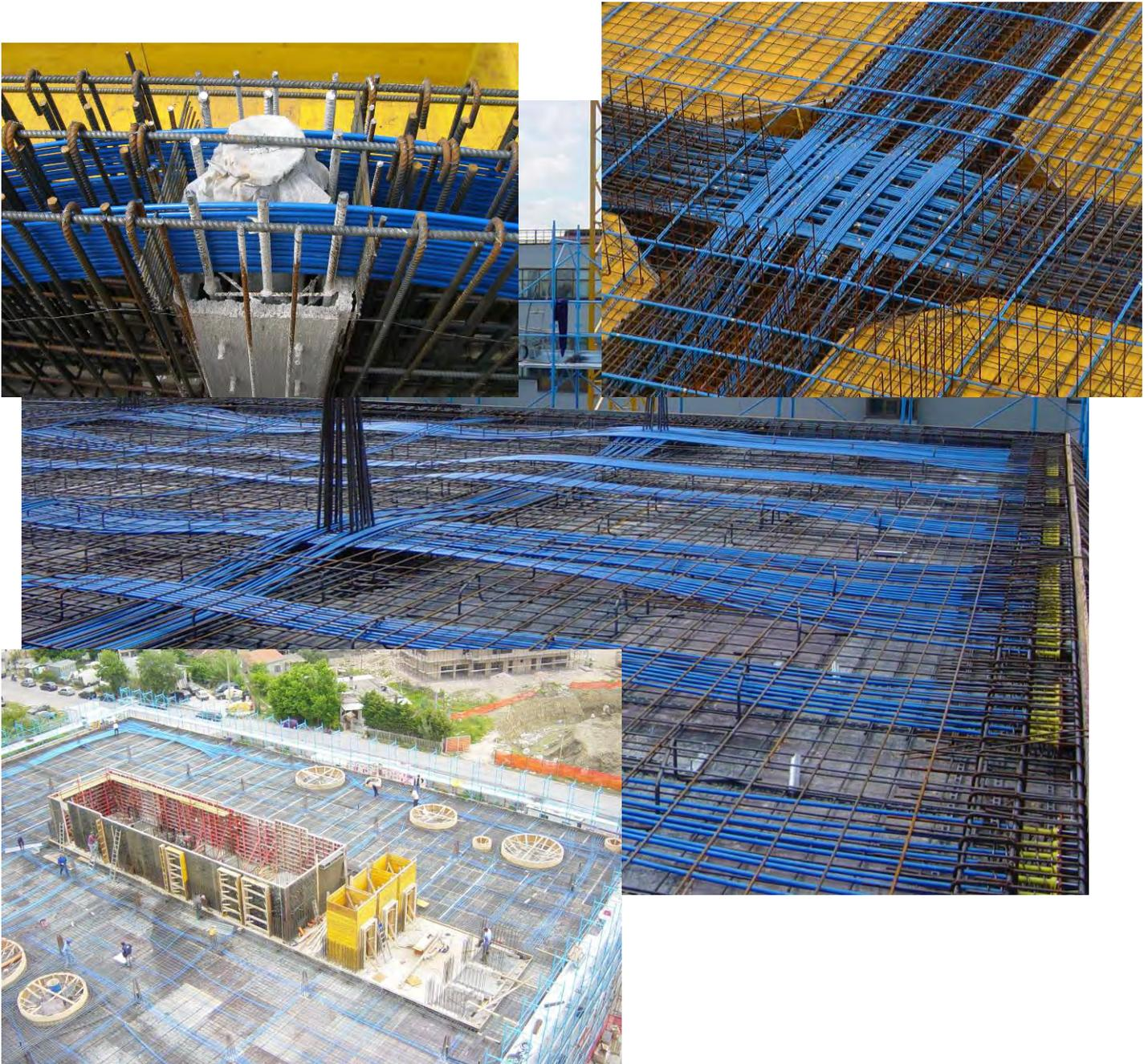
The use of post-tensioned concrete and, in particular, of concrete with unbonded cables requires to revise some long accepted principles of design.
